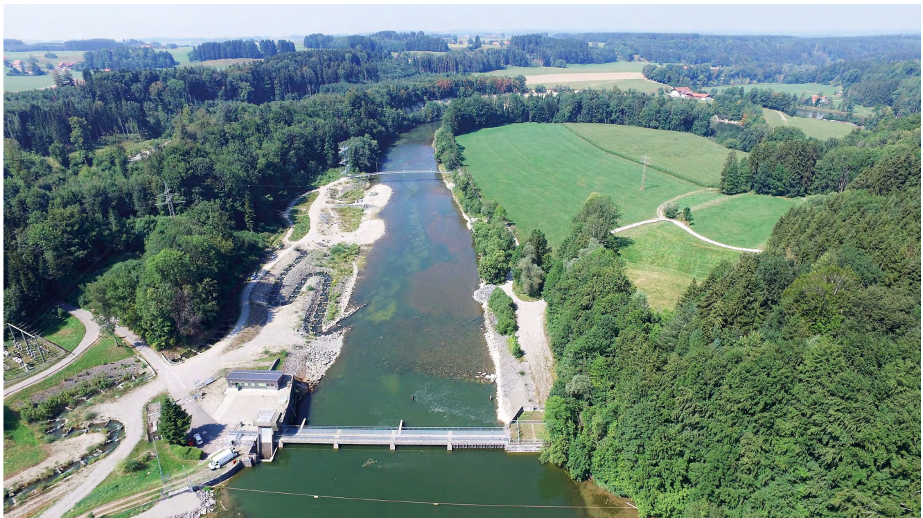
Figure 3: The hydropower plant 'Illerstufe 6' near Legau. The fish-bypass channel at the left shoreline is clearly visible. There have been bed load additions at the right shoreline and shore levelling at the left shoreline. At the midstream of the main riverbed, flat rock is visible as light ground. Credit: Olav König.
