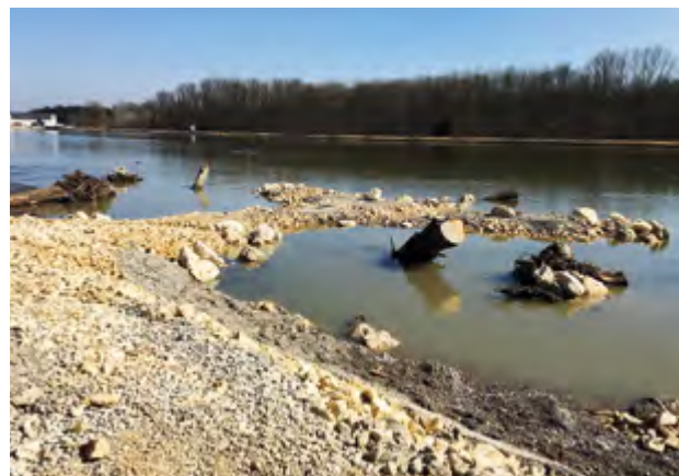
Figure 1. Installed 'eco-berm' at Offingen hydropower plant. On the opposite side there is still the traditional concrete embankment.
