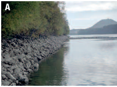
Figure 3. Riverbank restoration and rip-rap removal. A = typical rip-rap construction for river bank fixation. B = natural river bank with gravel bar after rip-rap removal. (Fotos: © viadonau)
