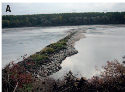
Figure 2. A = old groyne at low flow water level (LFW) +0.5 m. B = new groyne with declinant shape at LFW +0.3 m. In the front the lowered groyne base can be seen, which is now constantly overflown. (Fotos: © viadonau)
