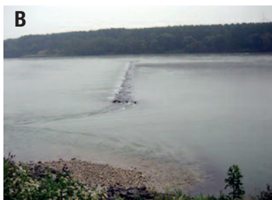
Figure 2. A = old groyne at low flow water level (LFW) +0.5 m. B = new groyne with declinant shape at LFW +0.3 m. In the front the lowered groyne base can be seen, which is now constantly overflown. (Fotos: © viadonau)
