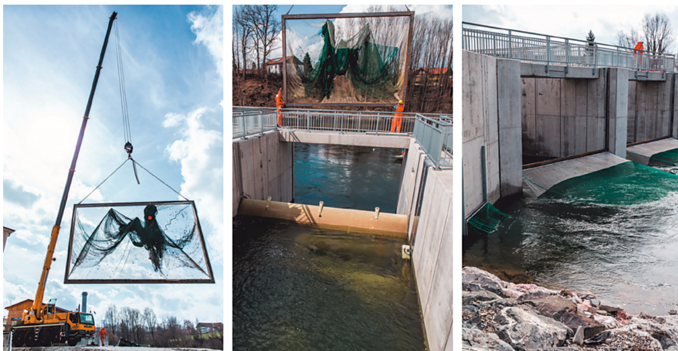
Figure 2: Setting up catch nets for investigating mortalities and fish injury patterns downstream of a hydropower plant. Photo credit: Martin Erd
