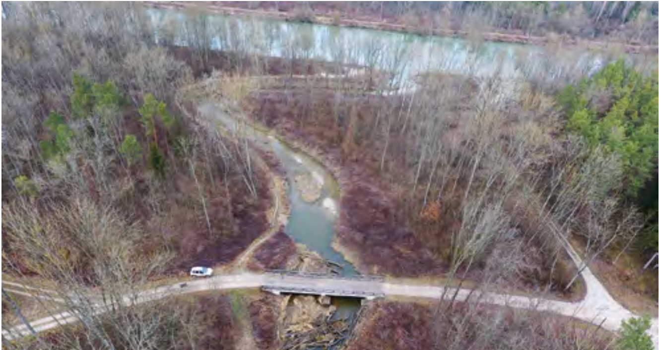
Figure 2. Stream reach from the bridge to the river mouth. Diverse instream structures and the new depositional gravel bars and the complex deadwood structure in front of the bridge, formed by the last flood event (photo P. Fischer).
