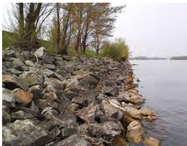
Figure 4. Riprap as it is found at most of the Danubian shoreline
