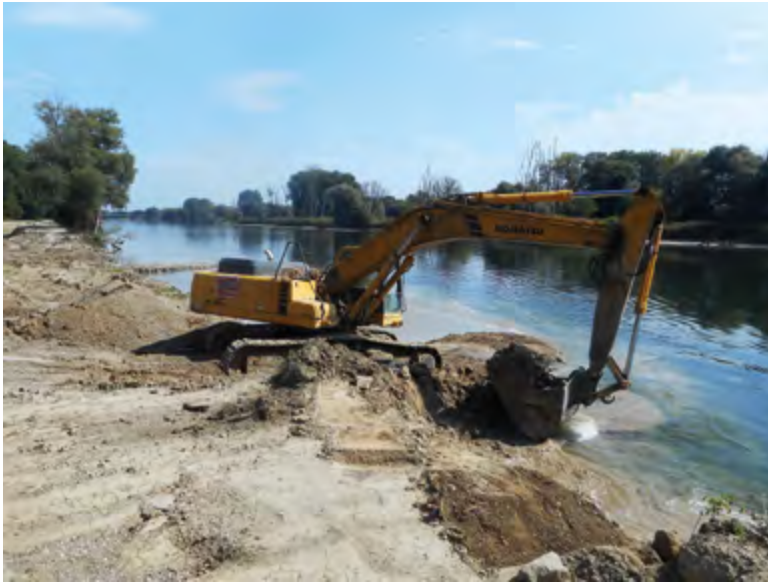
Figure 5. Removal of embankment and silt deposition by chain dredger
