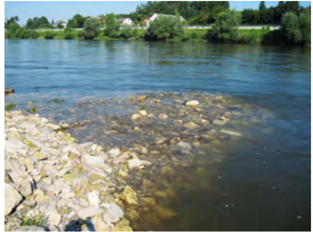
Figure 2. Steer groins using rocks from embankments, covered during medium discharge
