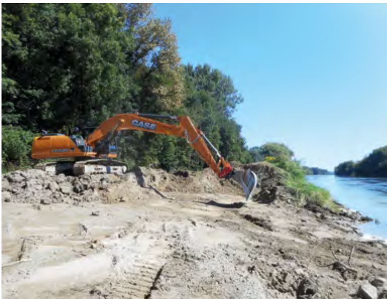
Figure 6. Shallow water zones with gravel banks
